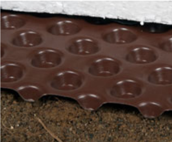
Drainage mats also provide a thermal break under the vapor barrier.
