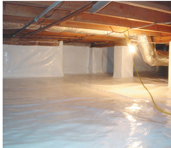
The entire crawlspace should be lined with vapor barrier, not just the floor.
